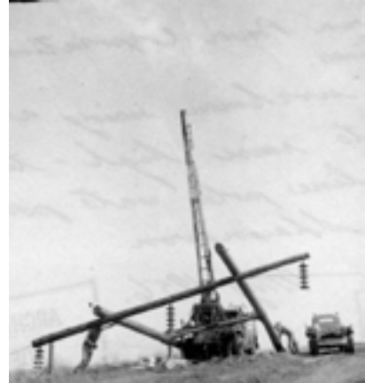
SaskPower Corp. workers raising high-tension power line poles into position near Shaunavon, SK, 1956. Saskatchewan Archives Board R-A13087(1)
