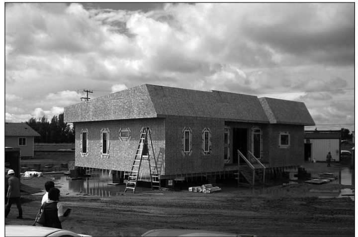
VerEco home under construction in Vanscoy, August 2010.
